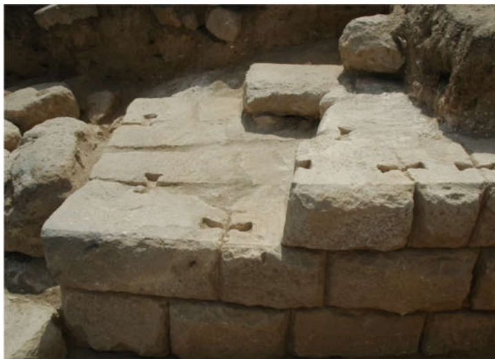
Fig 06 – The dovetailed interlocking system for the stone slabs
